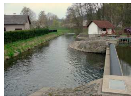
Letohrad Small Hydroelectric Power Plant
