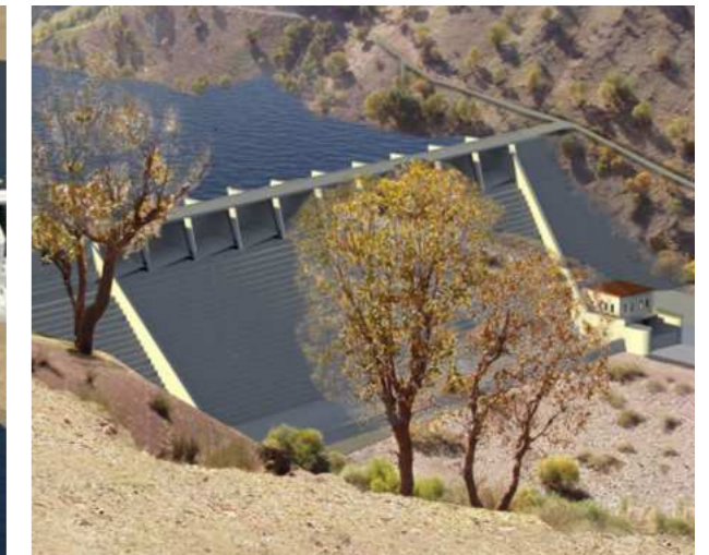
Design of the Quatabian Dam in Sulaymaniyah
